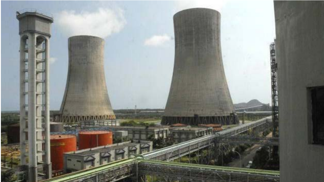
Figure 2. Hyperboloid Cooling Towers installed in a thermal Power Plant
